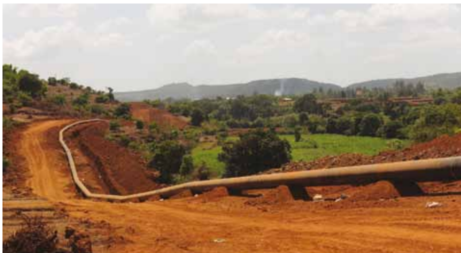
Preparing to lower in the Dabhol – Bangalore Pipeline.
