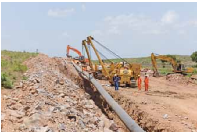
Figure 2. Lowering of pipe.
