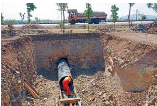
Figure 3. Boring work underground.
