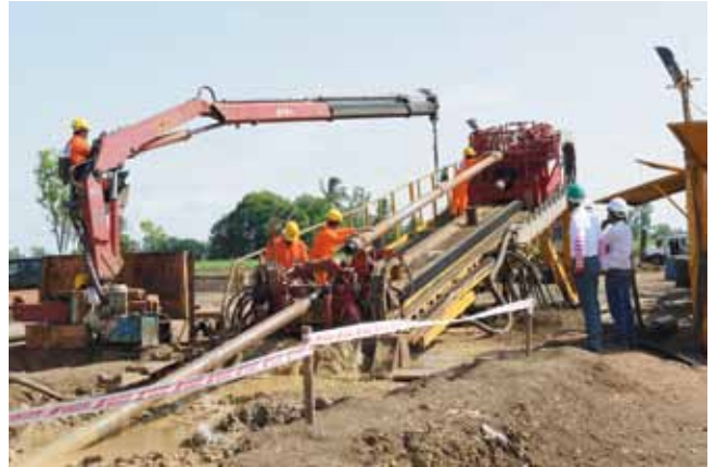
Figure 4. HDD in progress.
