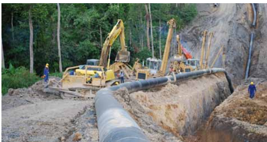
Preparing to lower-in the SSGP.
