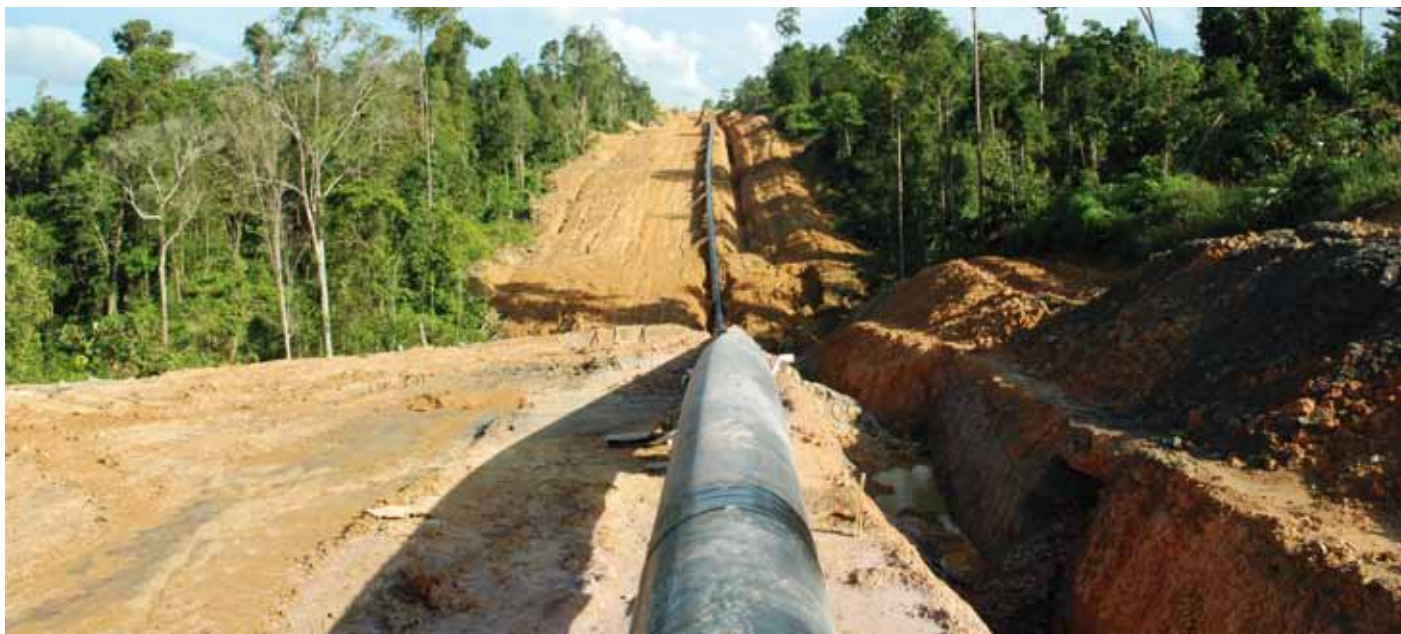
The welded pipeline alongside the trench.
